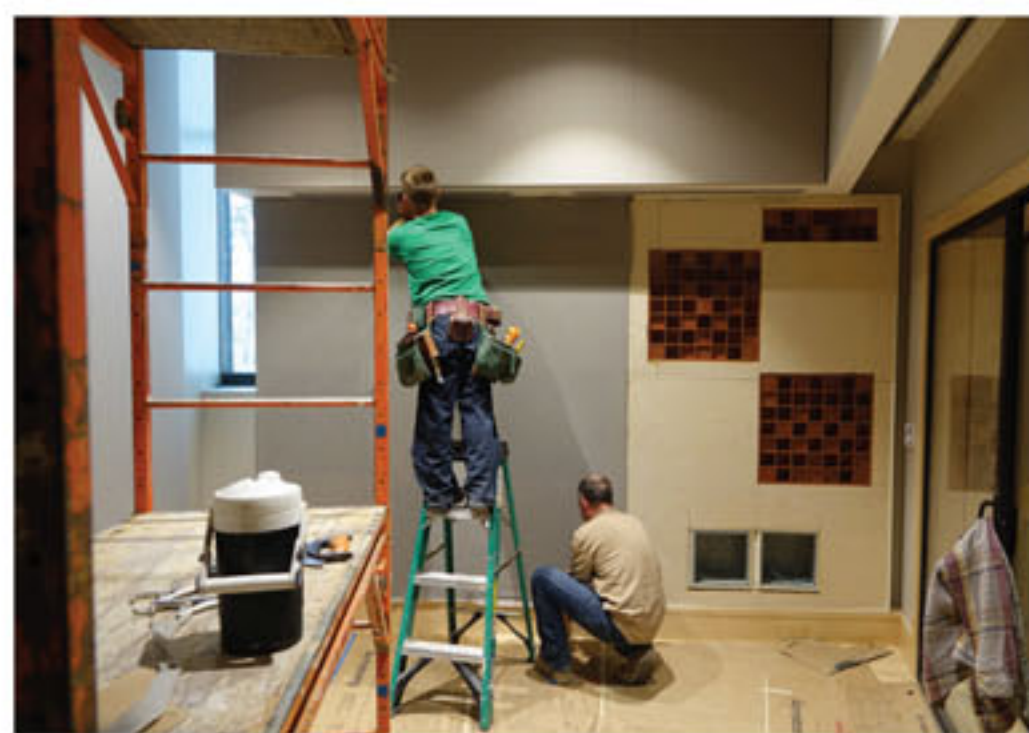
Treatment in the piano iso booth includes alternating squares of absorption and diffusion, clouds in the ceiling, and a slice of natural light.
